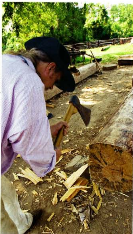
Toppling a tree and stripping it of its limbs and bark is hard enough, but shaping the log by hand for building takes several more hours, as Colonial Williamsburg carpenter Corky Howlett demonstrates.
